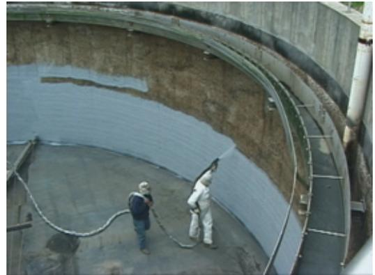
**DISCUSSION:** Badly eroded eight year old concrete walls and floor of primary clarifier in food processing plant were severely weakened and in danger of failure. The owner had tried epoxy lining which had failed in three years. It was decided to re-line with WARRIOR™ 260 which would stand up to the high concentration of calcium sulfate chemical used.
