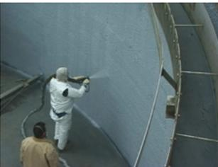
All surfaces were sand blasted cleaned, followed by sprayed primer coat of Pronto Prime concrete priming lacquer. Topcoat of .080 inch thick WARRIOR™ 260 was applied. Entire job was completed in 24 hours and re-watered in two hours.
