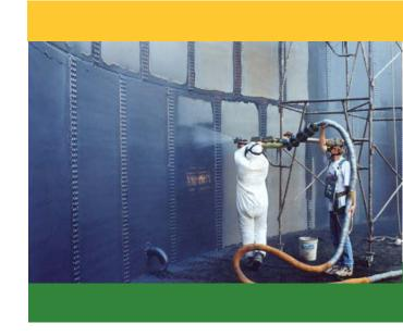
The steel surface was badly contaminated with dissolved chlorides as might be expected. The dissolved salts were removed to a level of 20 ug / cm² with a proprietary cleaning chemical and process. The steel was coated with .080 inch thick POLYARMOR® 80-775 prior to blush set in on the steel surface.
